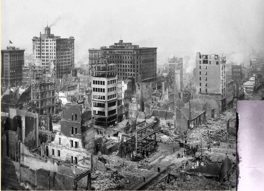
14. San Francisco earthquake damage near Post and Grant Avenues.
